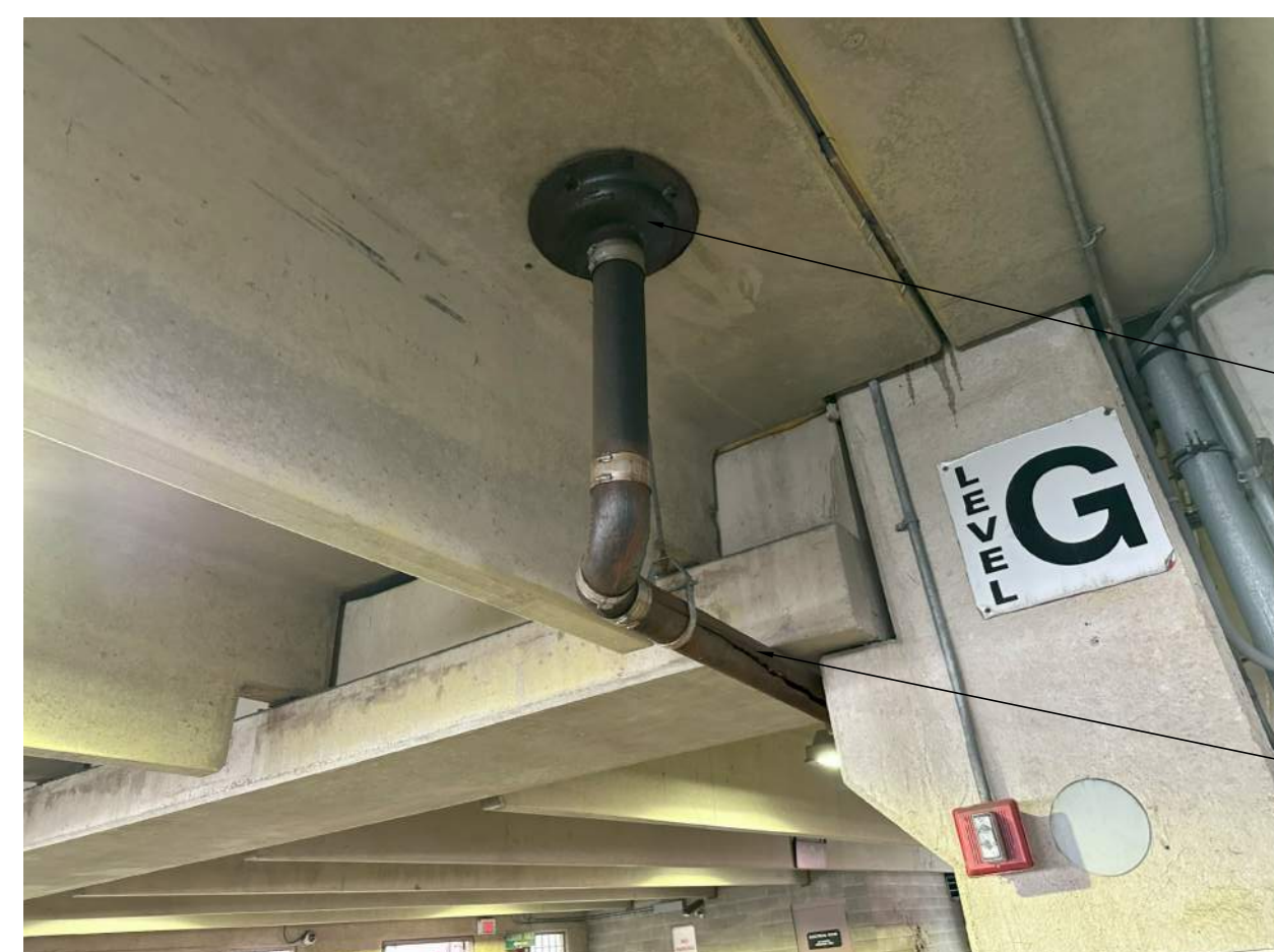
TYPICAL DRAIN & DRAIN LINE REPLACEMENT DETAIL
